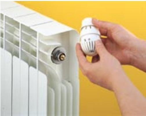
Aprire completamente la testa portando la manopola in posizione
