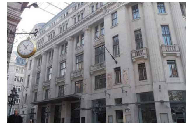
LOCATION: HUNGARY - PROJECT: SHOPPING CENTER
