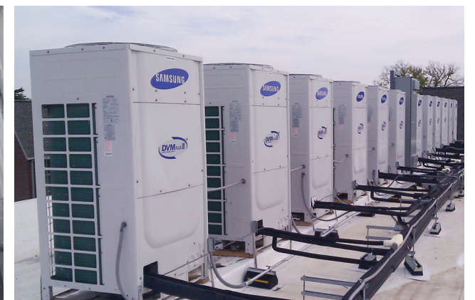
LOCATION: TENNESSEE, USA - PROJECT: LIPSCOMB COLLEGE
